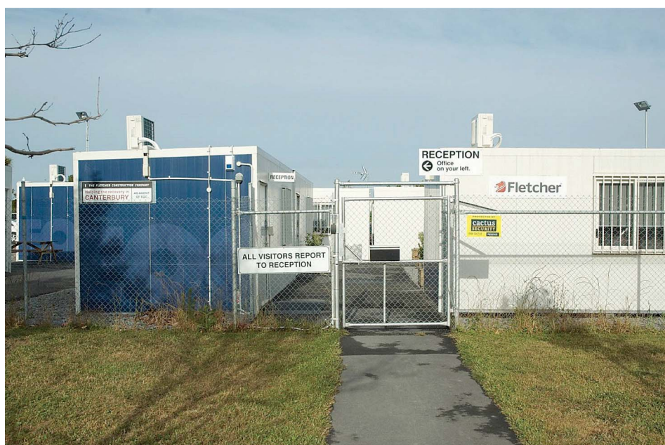
Figure 2 Picture of a typical repair hub
